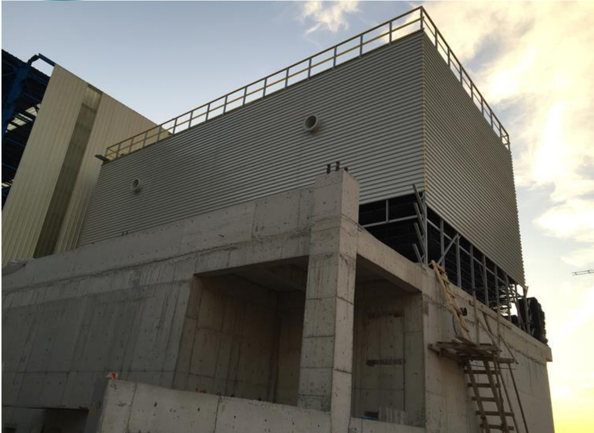
Cooling Tower Installation
