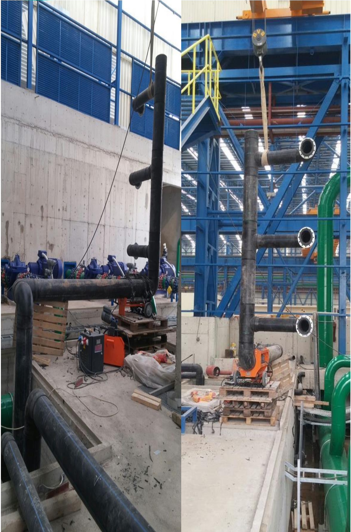
Pump Discharge Line (PE100 HDPE Pipe) Installation
