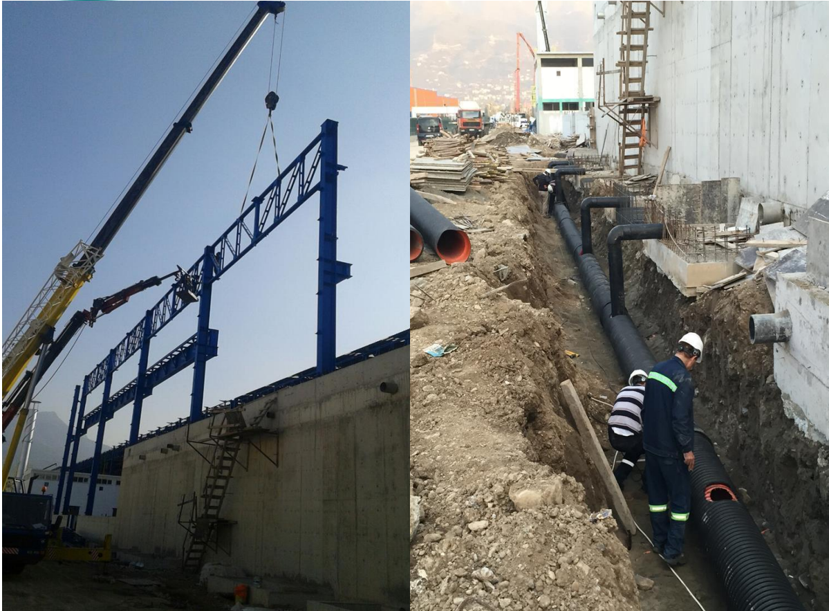
Process Water Treatment Basins Drain and Overflowing Installation
