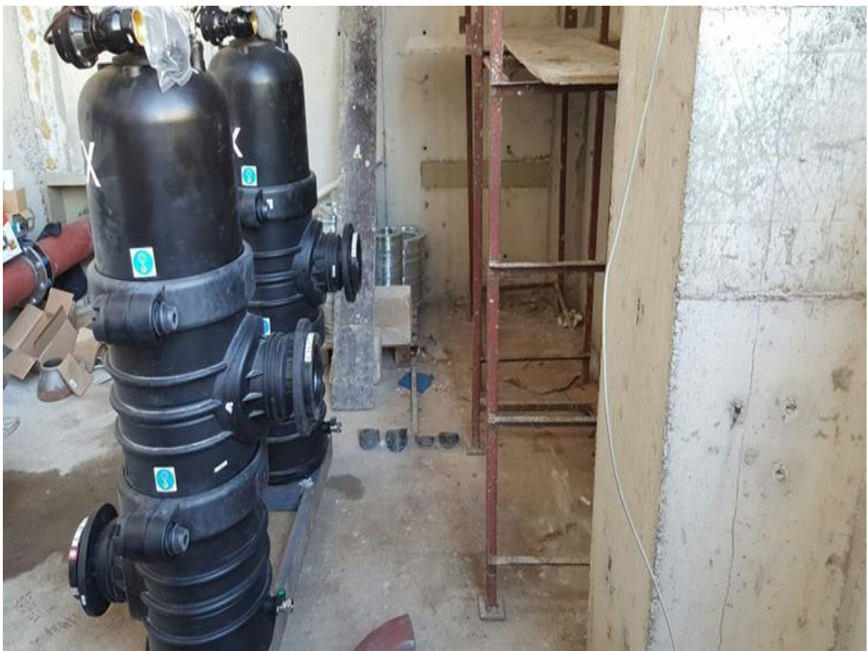
Circulation System with Side Stream Filters Installation
