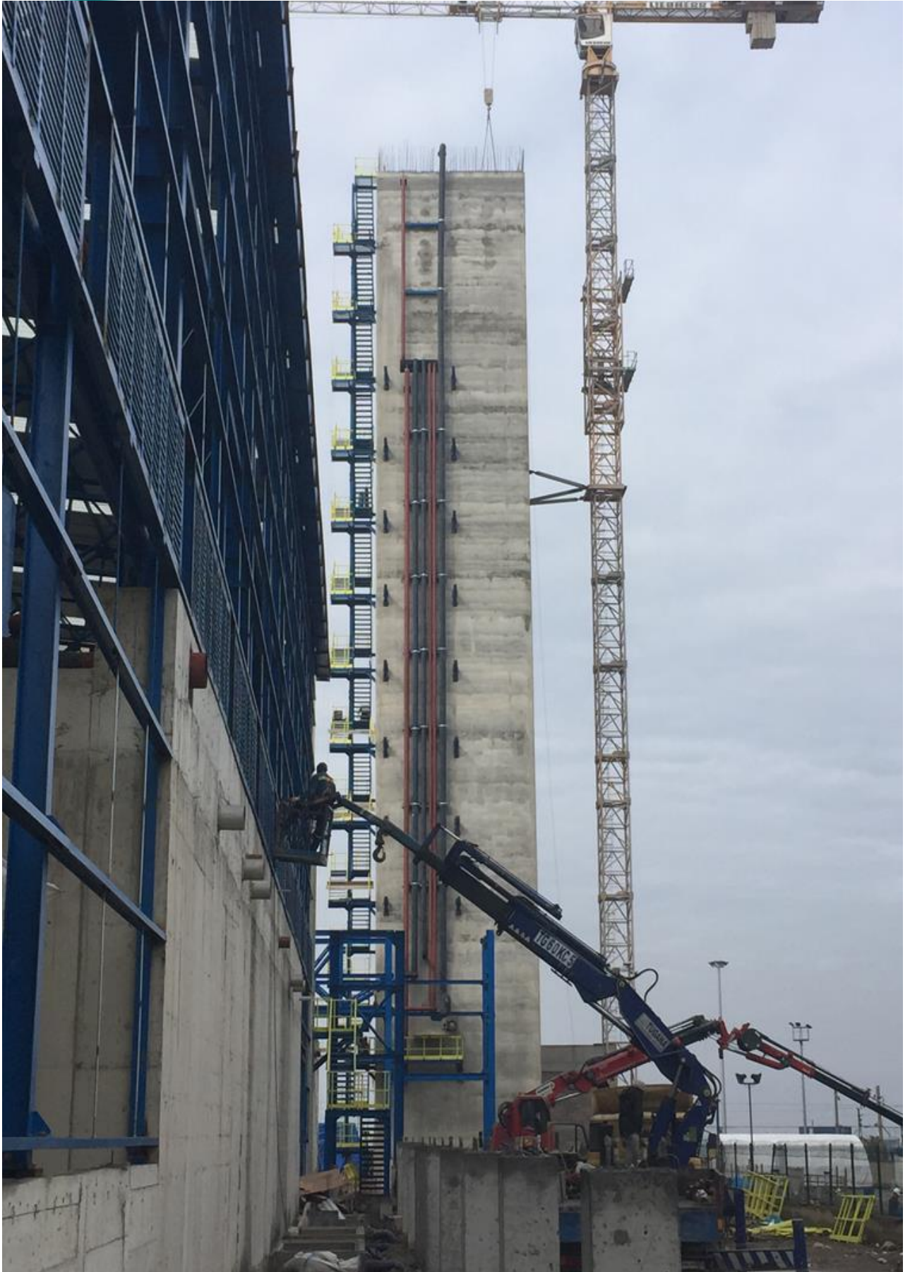
Process Water And Emergency Water Basin Tower Pipeline Installation
