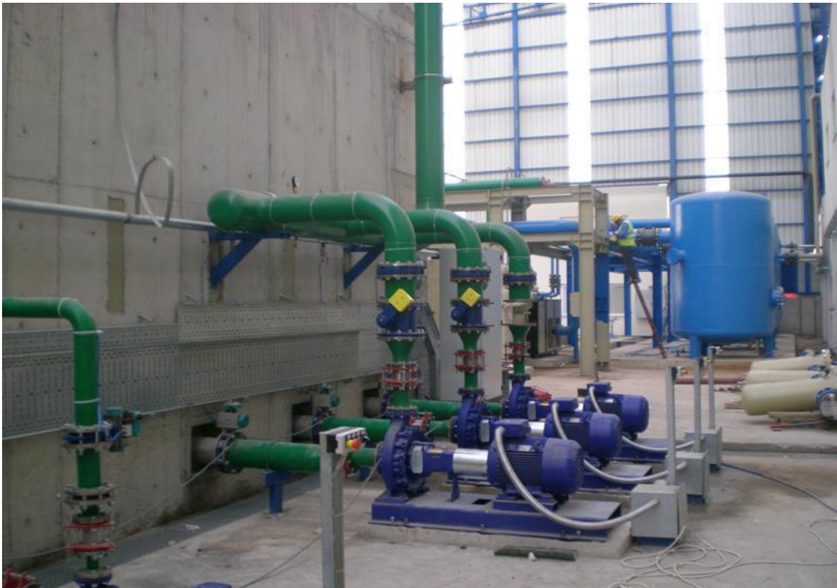
Sand Filter Pumps And Compressed Air Tanks Installation
