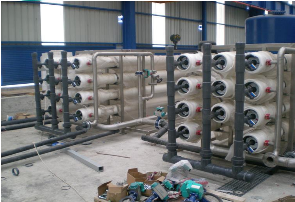
Reverse Osmosis Pure Water Line Installation
