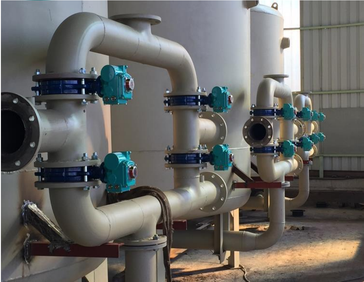
Sand Filter Valve Installation
