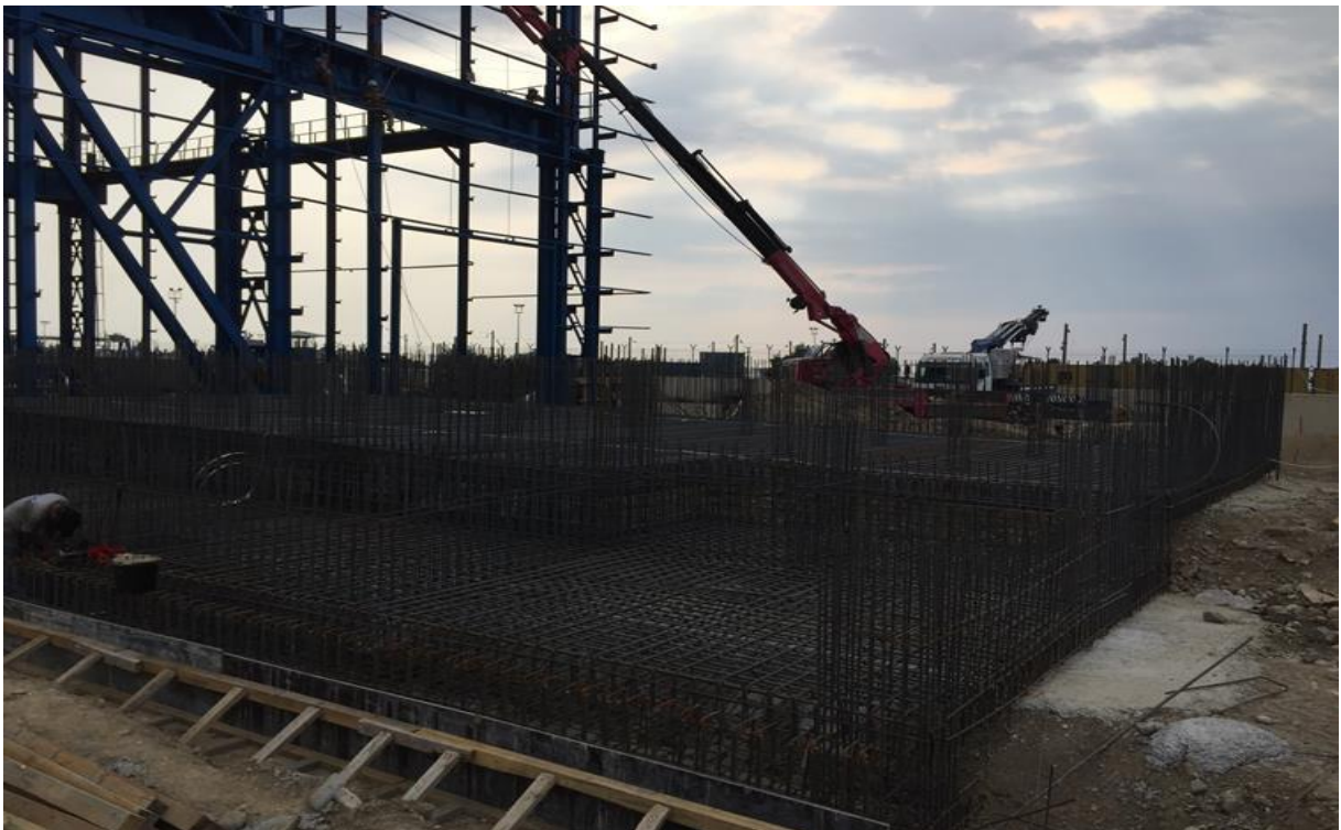
Pumps Suction and Water Basin Construction
