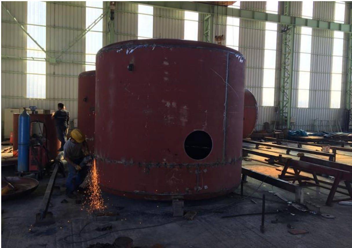
Sand Filter Installation
