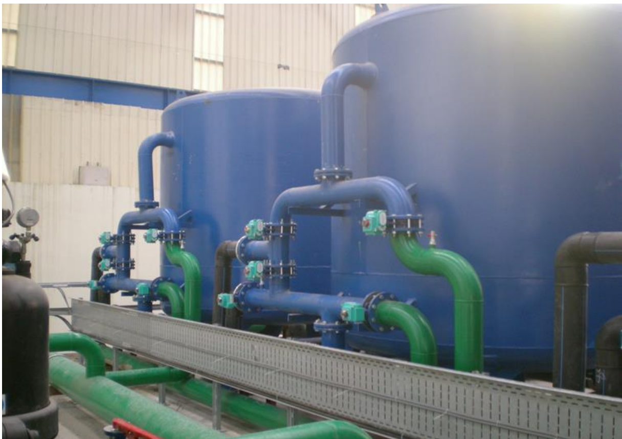
Sand Filter Installation
