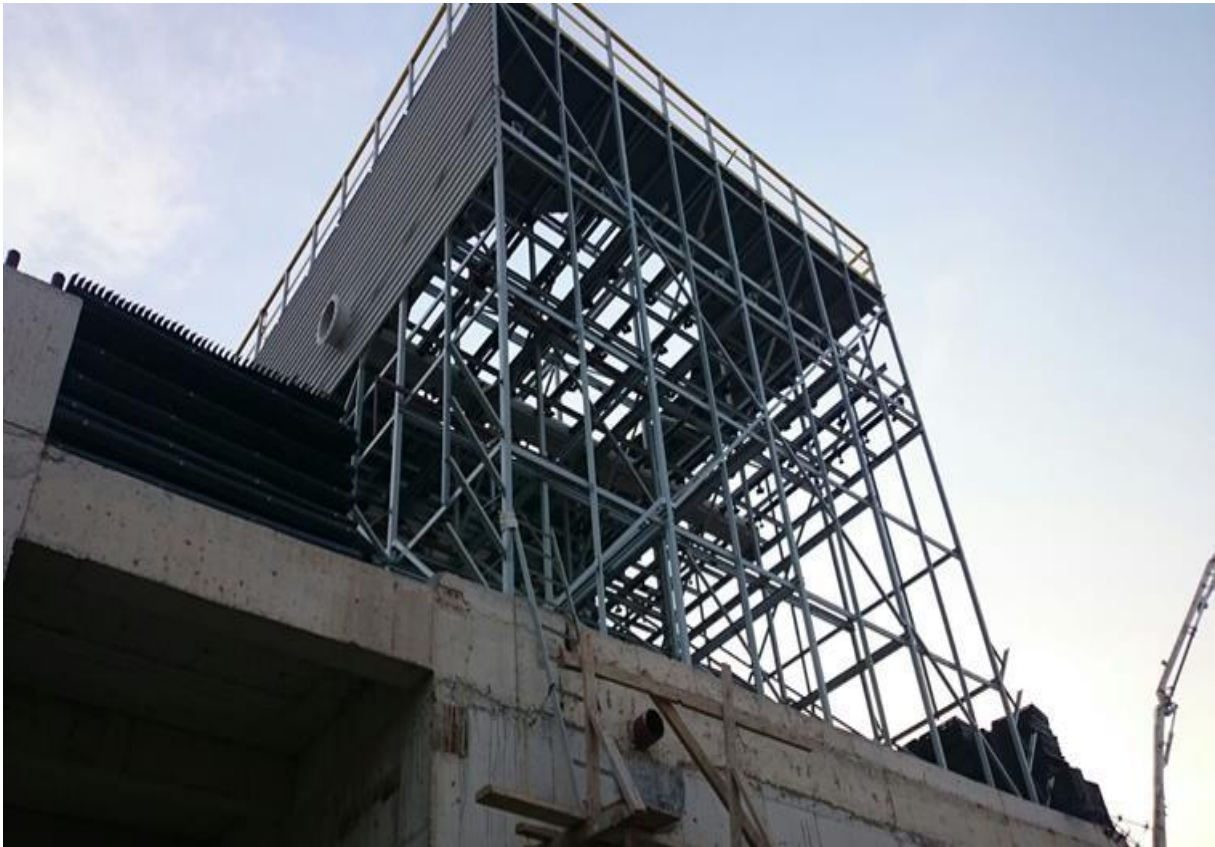
Cooling Tower Installation
