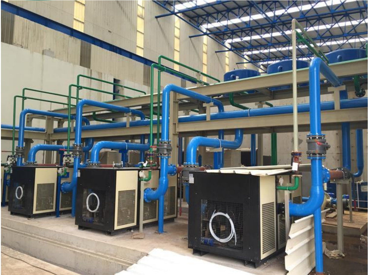
Compressed Air Plant Compressors and WTP Sand Filters (Upside) Installation
