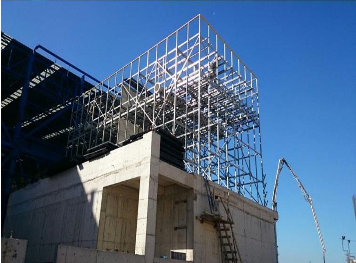
Cooling Tower Basin and Installation
