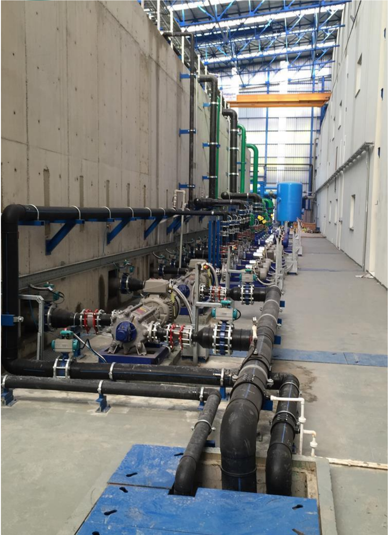
Process Water Treatment Pumps Installation
