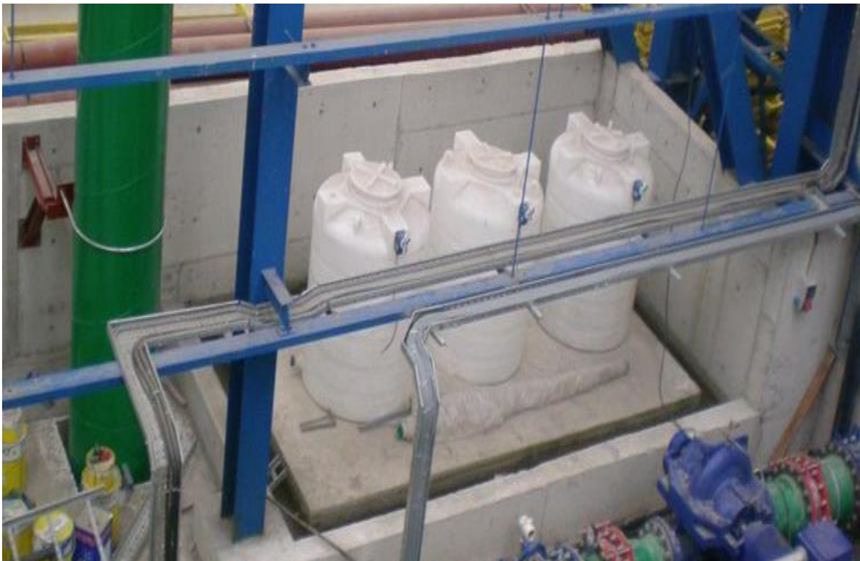
Circulation System Chemical Dosing Unit Installation
