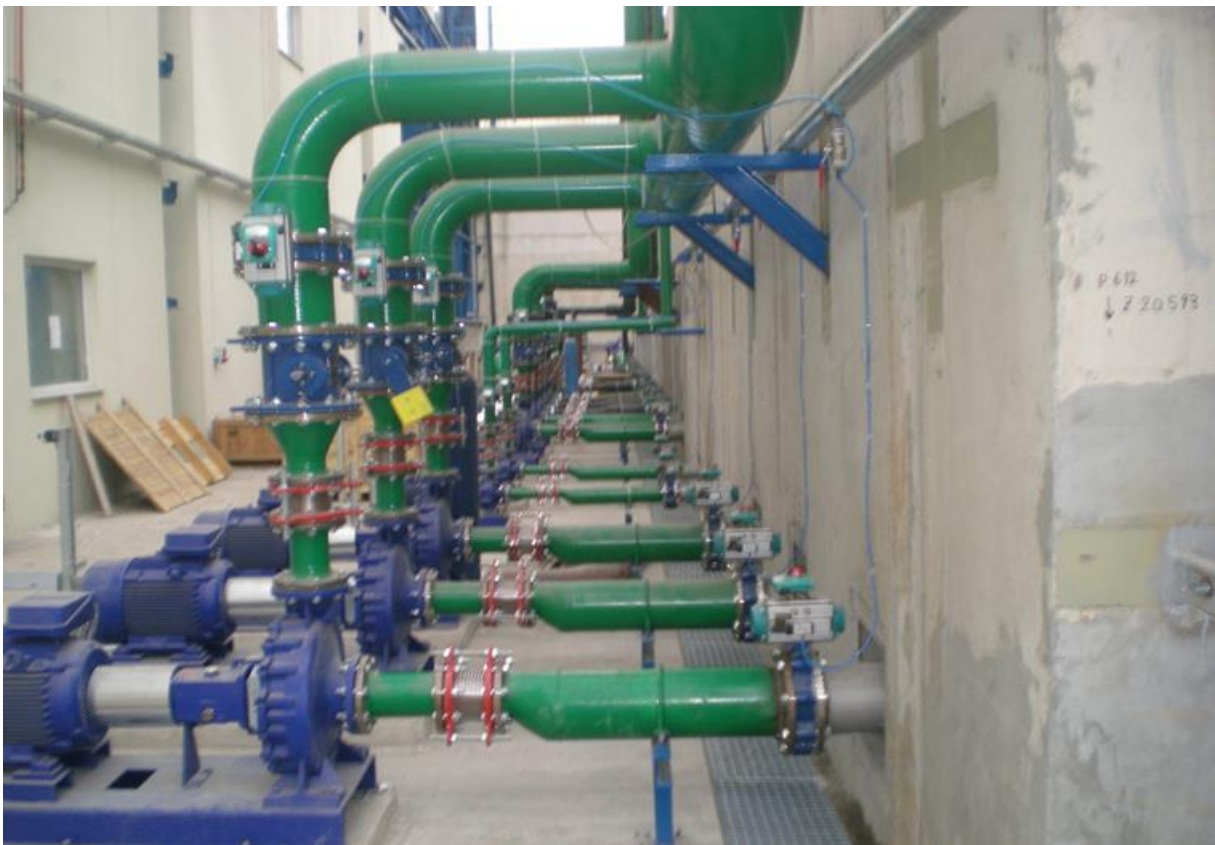
Process Water Treatment Pumps Installation
