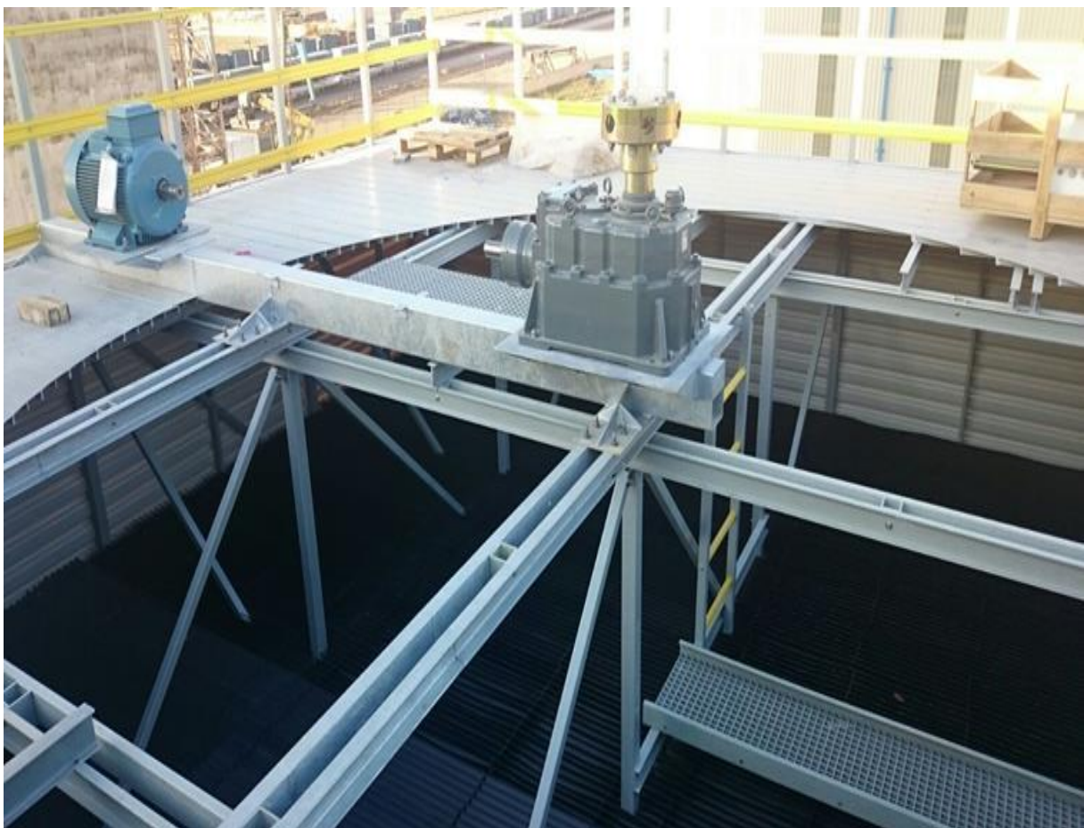
Cooling Tower Fan Installation
