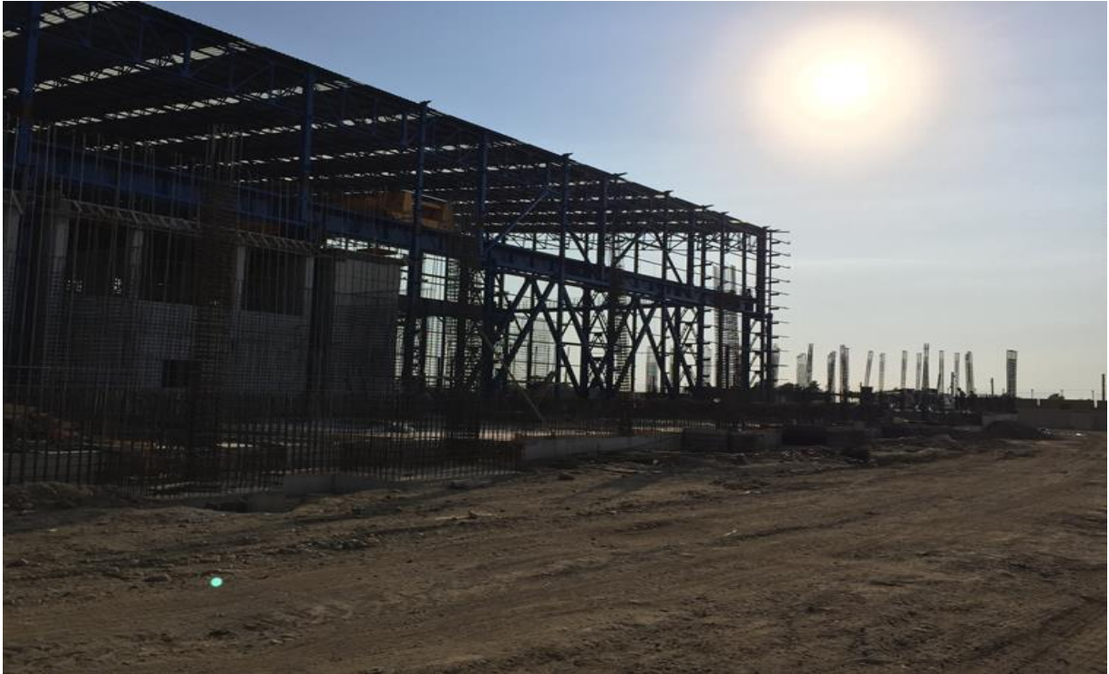
WTP Area Construction
