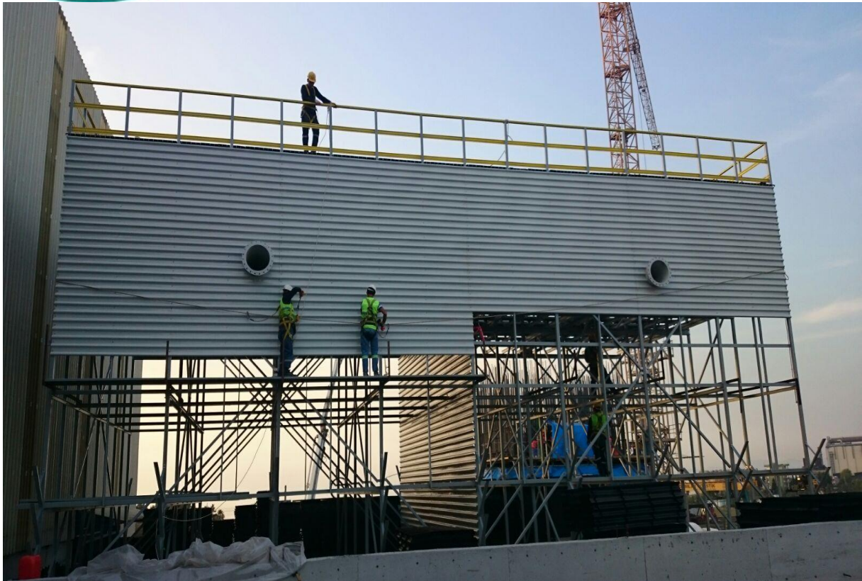
Cooling Tower Installation
