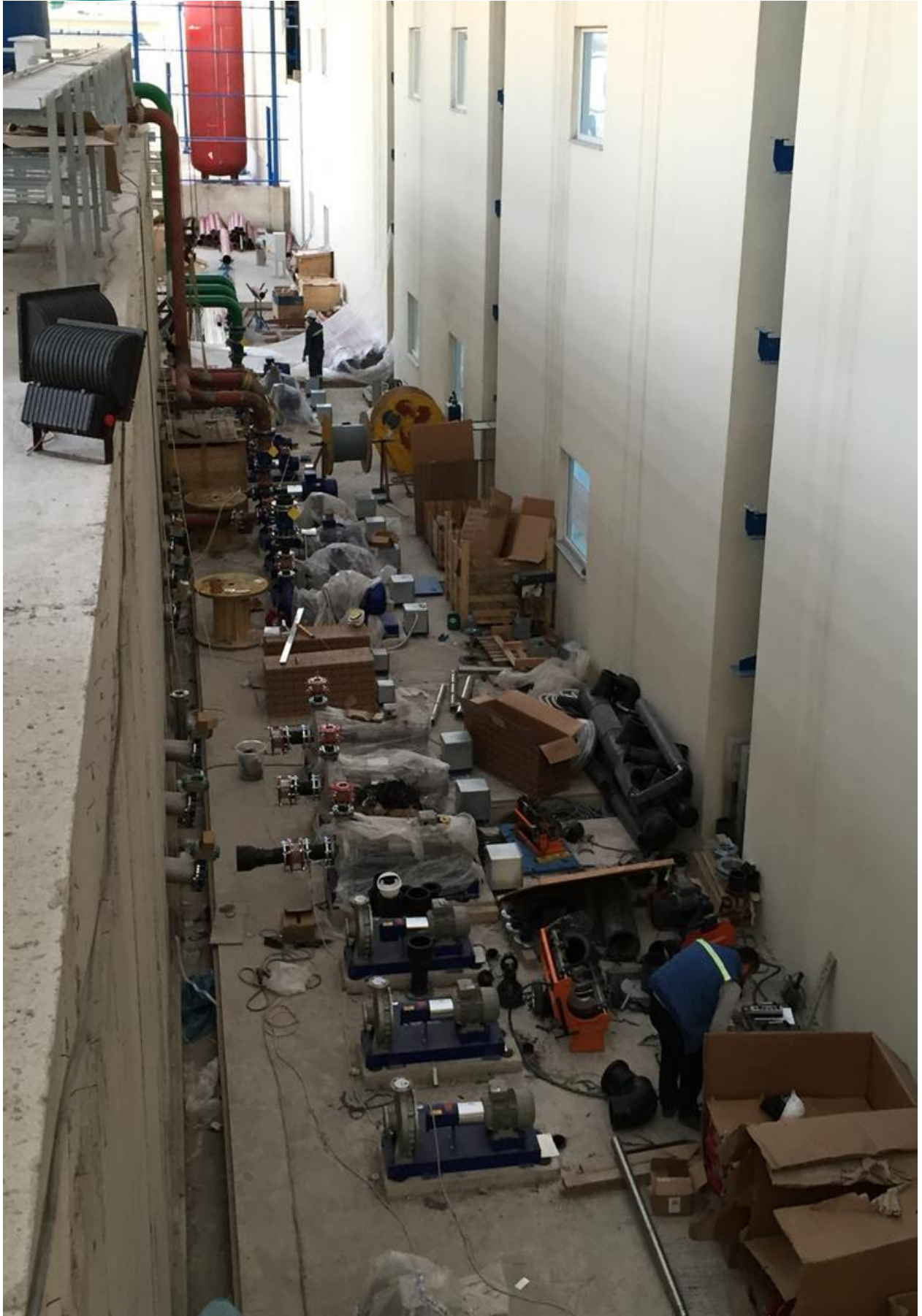
Process Water Treatment Pumps Installation
