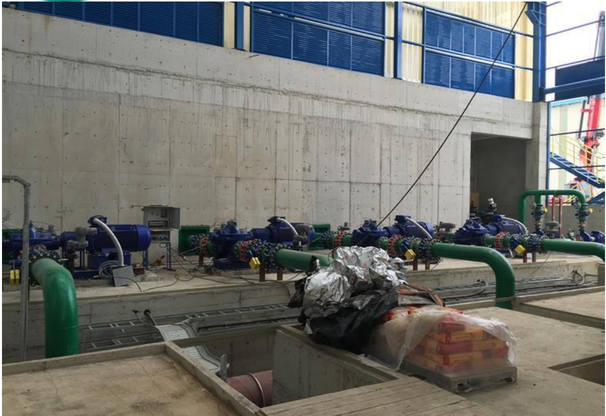
Circulation Pumps Installation
