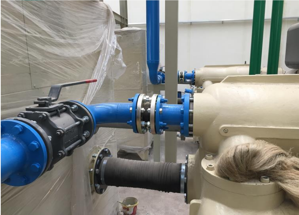
Compressed Air Plant Compressor Pipeline Intallation
