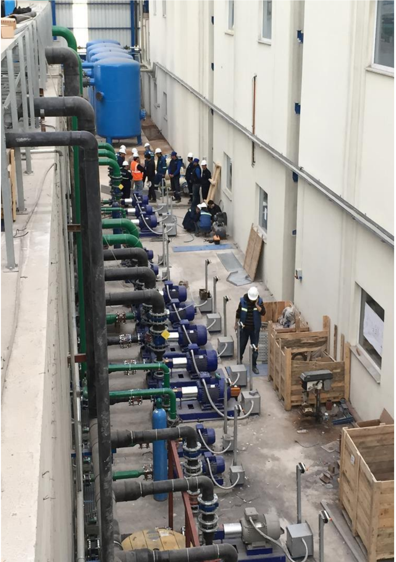
Process Water Treatment Pumps Installation
