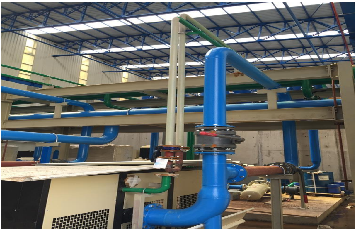
Compressed Air Plant Compressor Pipeline Intallation
