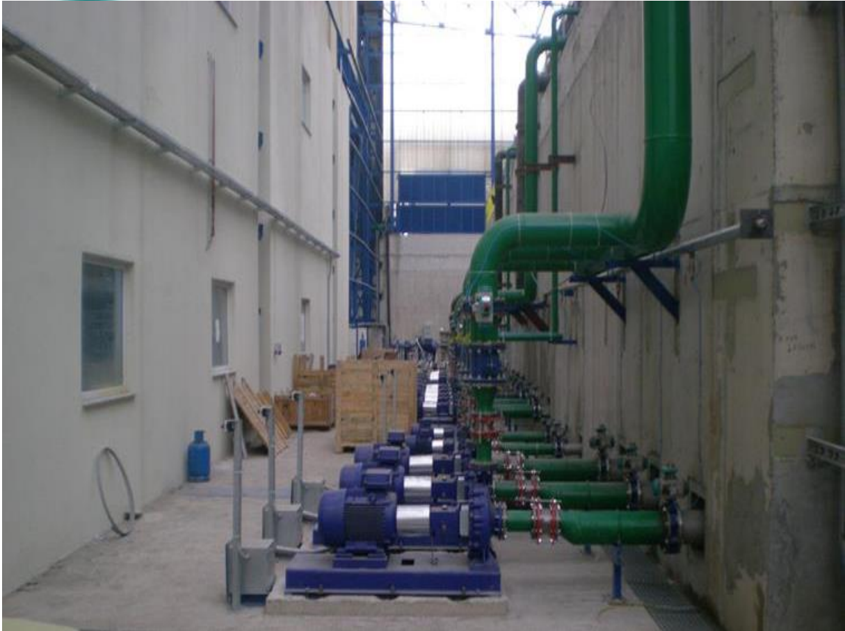
Process Water Treatment Pumps Installation
