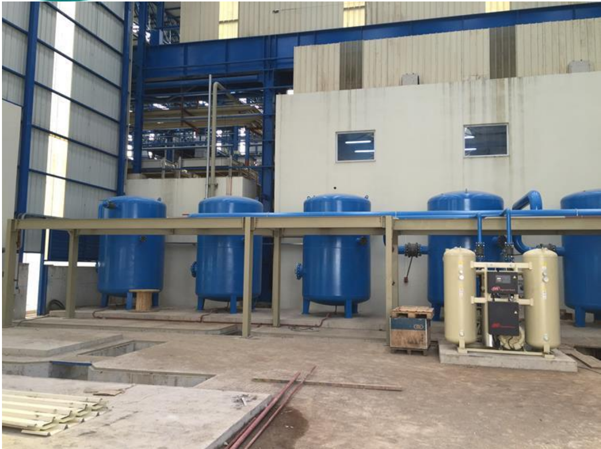
Compressed Air Plant Air Tanks and Pipeline Installation
