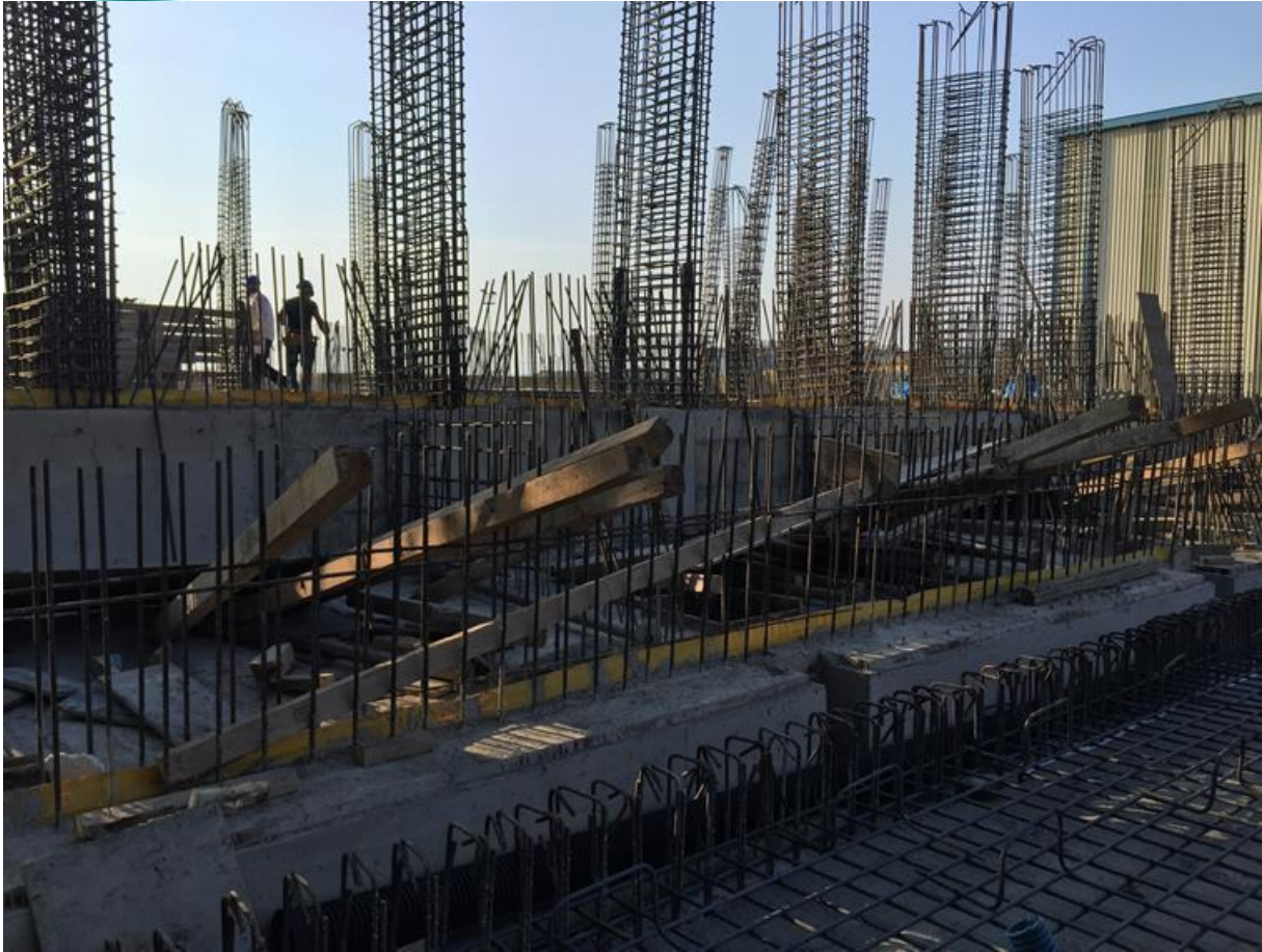
Cooling Tower Basin and Pump Suction Construction
