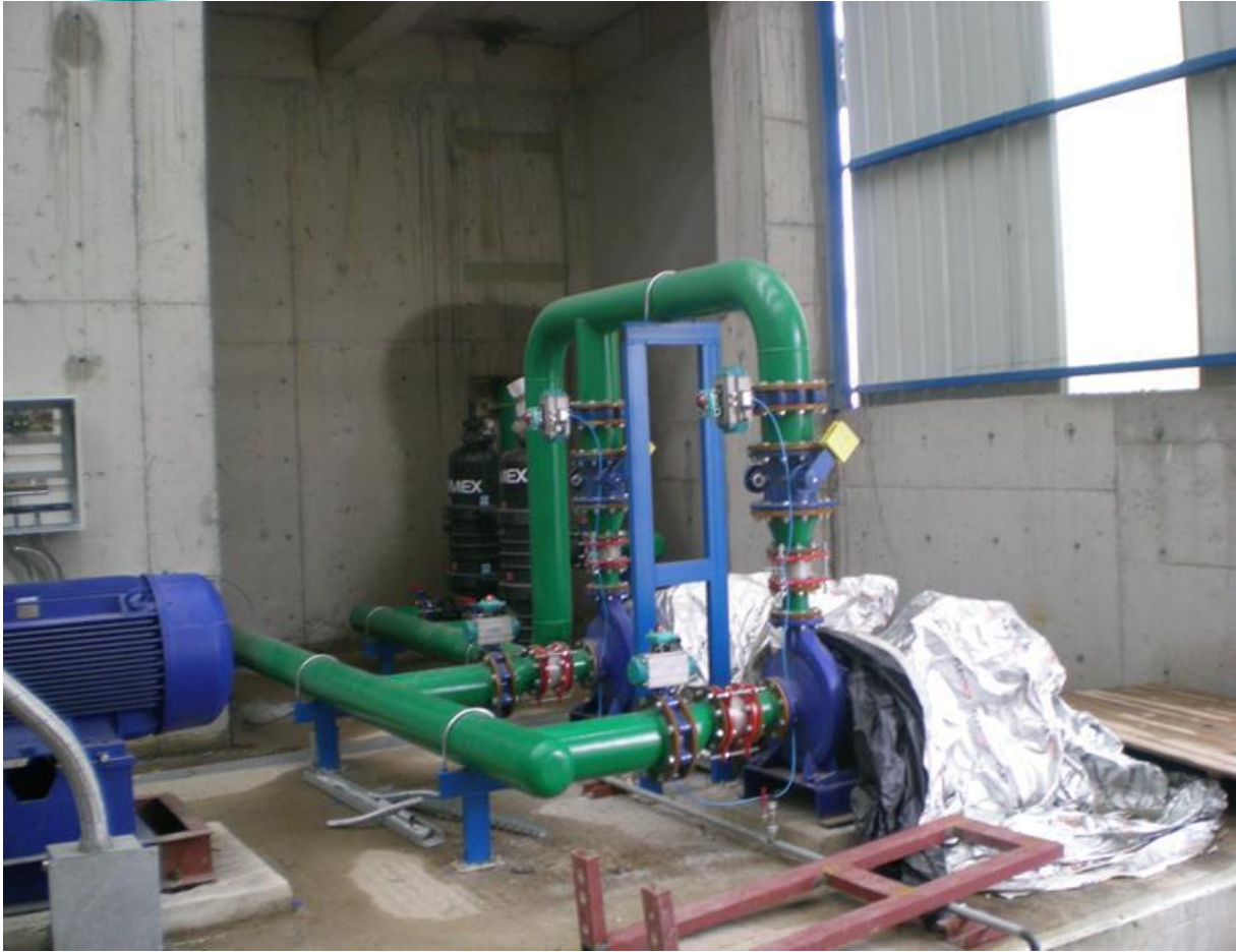
Circulation System with Side Stream Pumps and Filters Installation
