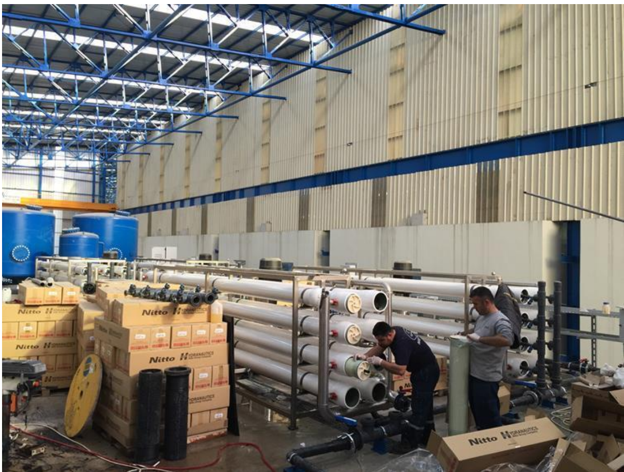
Reverse Osmosis Membrane Filter Installation
