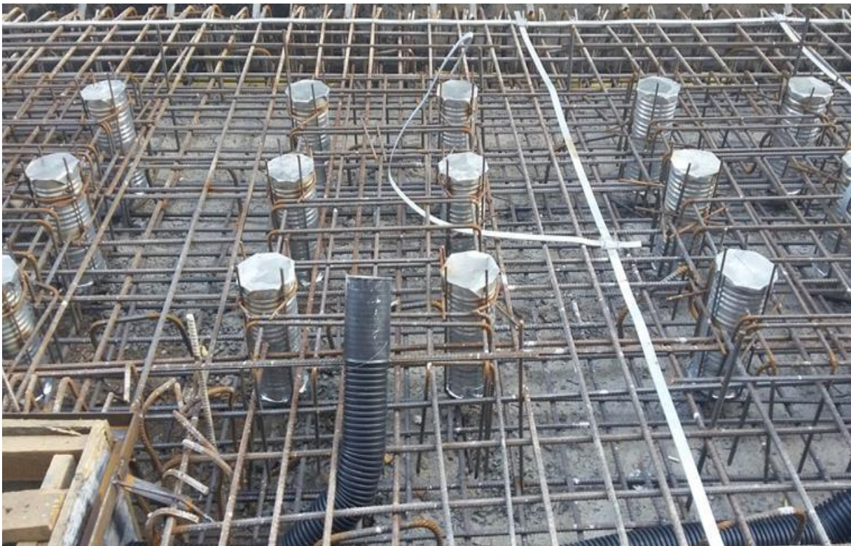
Pumps Anchor Embedded Area
