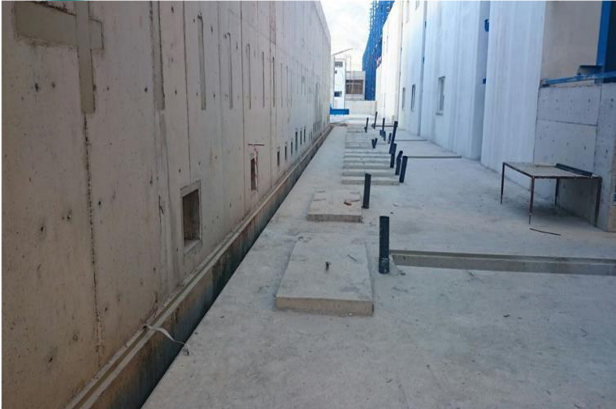
Pumps Suction Embedded Plates/ Pipeline Embedded Plate /Consruction/Electric Power Conduits
