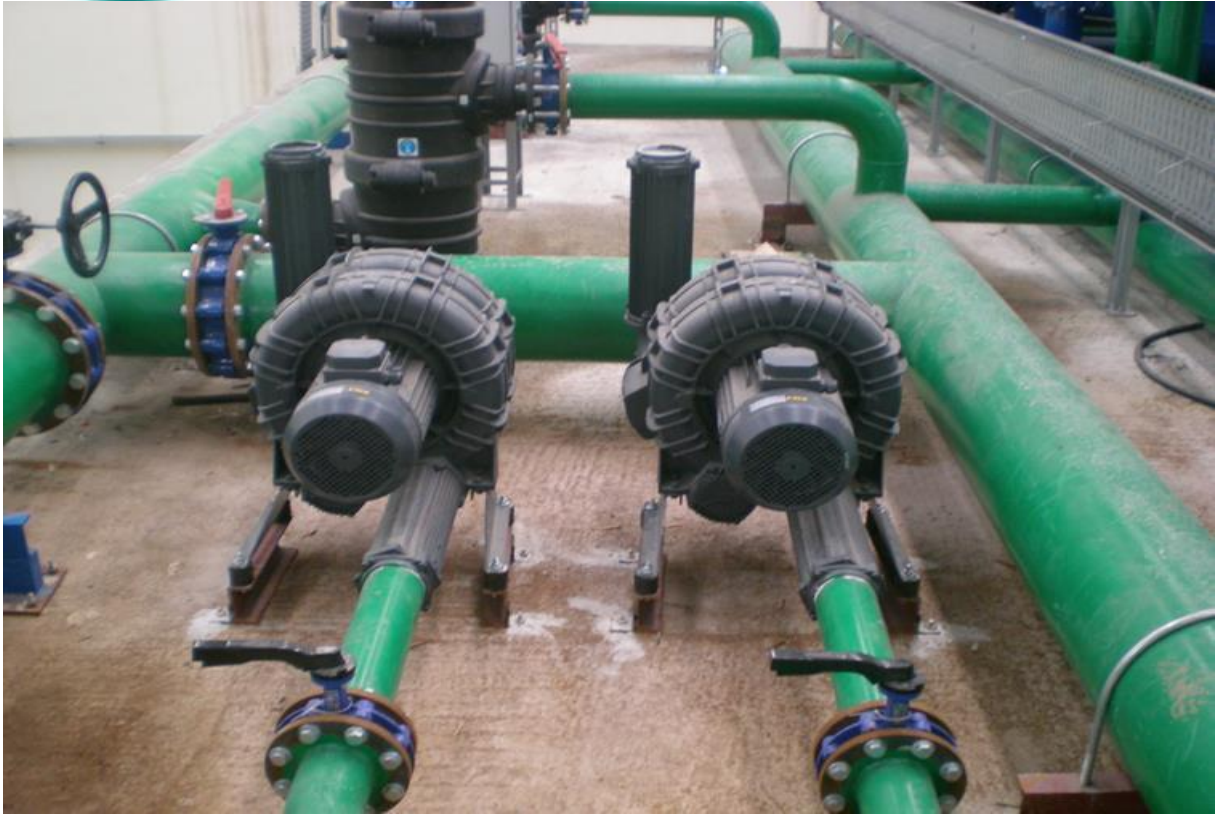
Sand Filter Blower Installation
