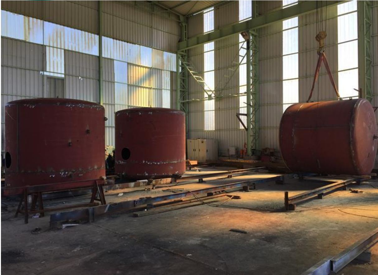
Sand Filter Installation
