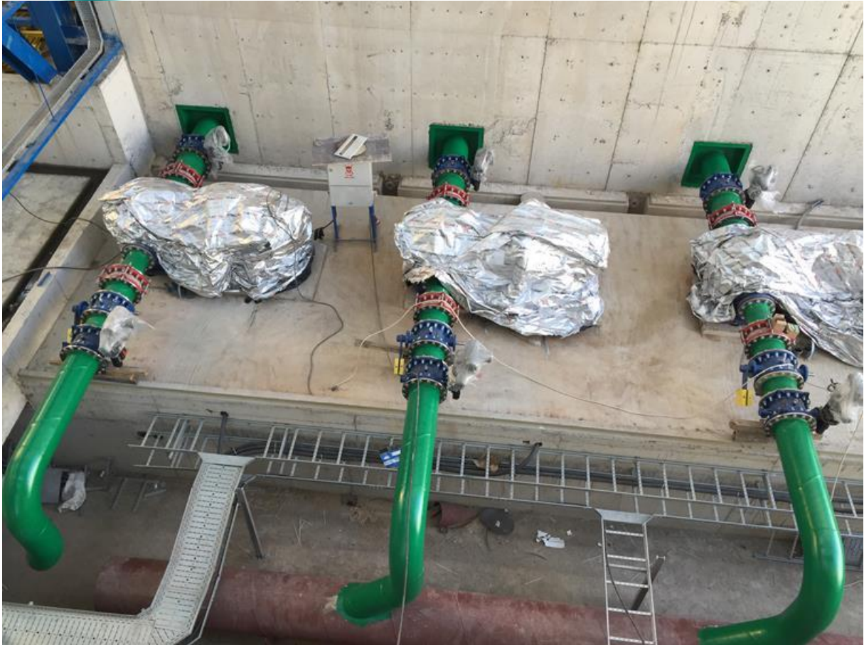
Circulation Pumps Installation
