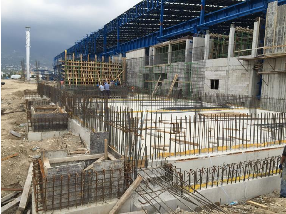
Water Basin Area Construction
