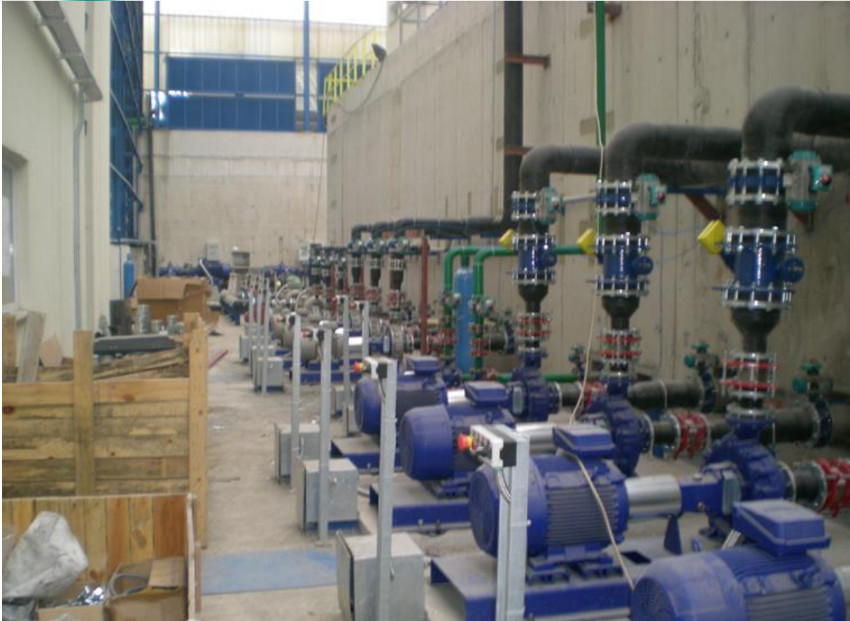
Process Water Treatment Pumps Installation
