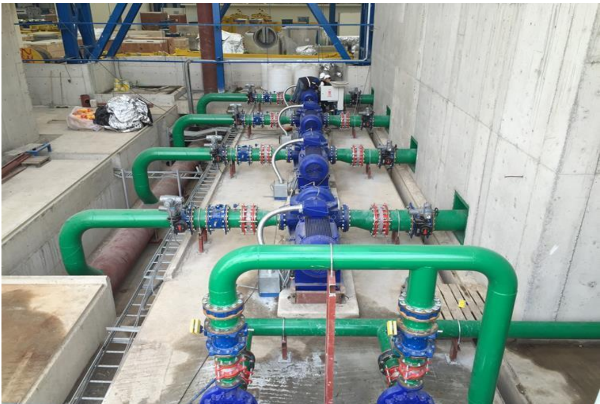
Circulation Pumps Installation
