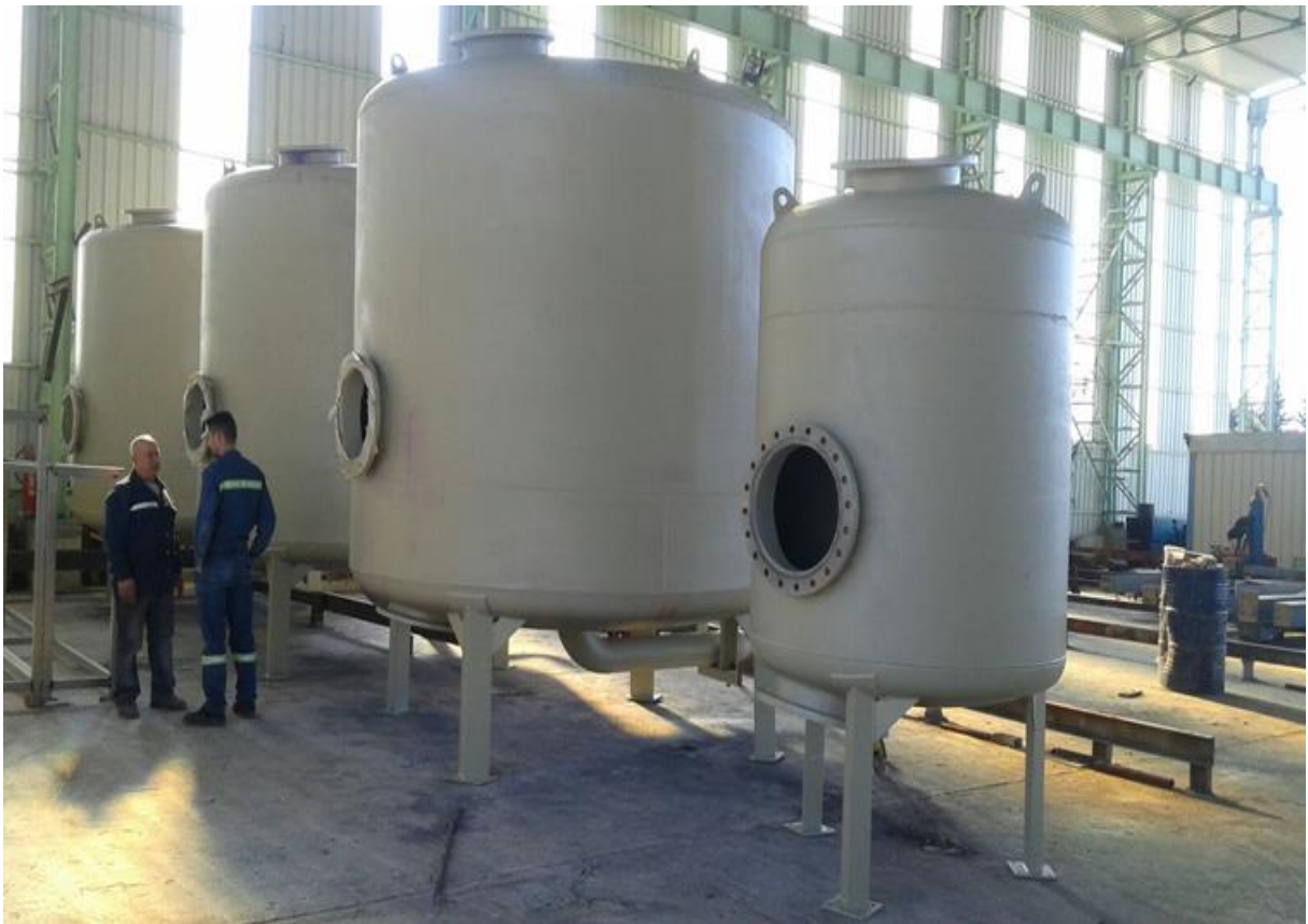
Sand Filter Installation
