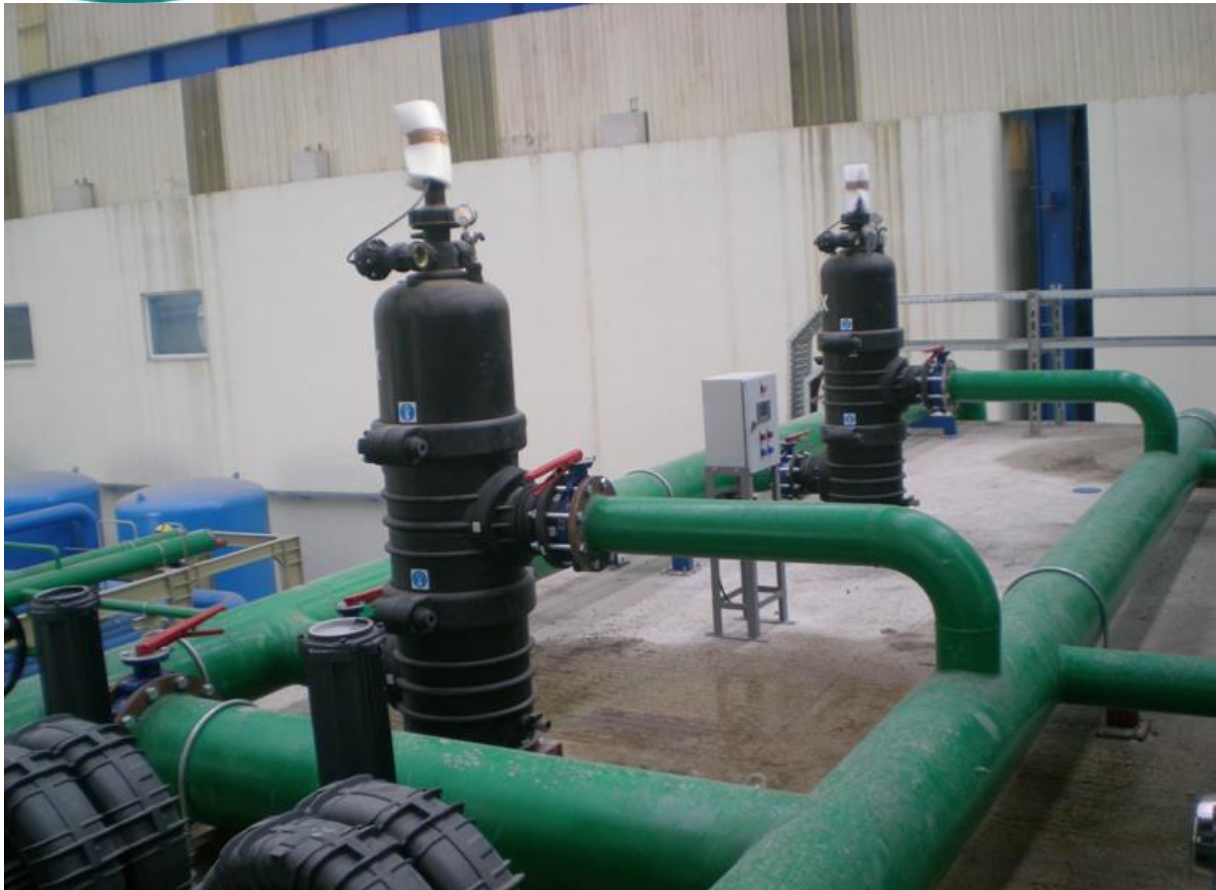
Process Water Mechanical Filters Installation
