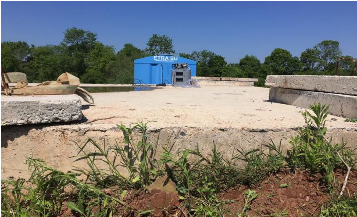
Wastewater Treatment Plant Sample and Discharge Point
