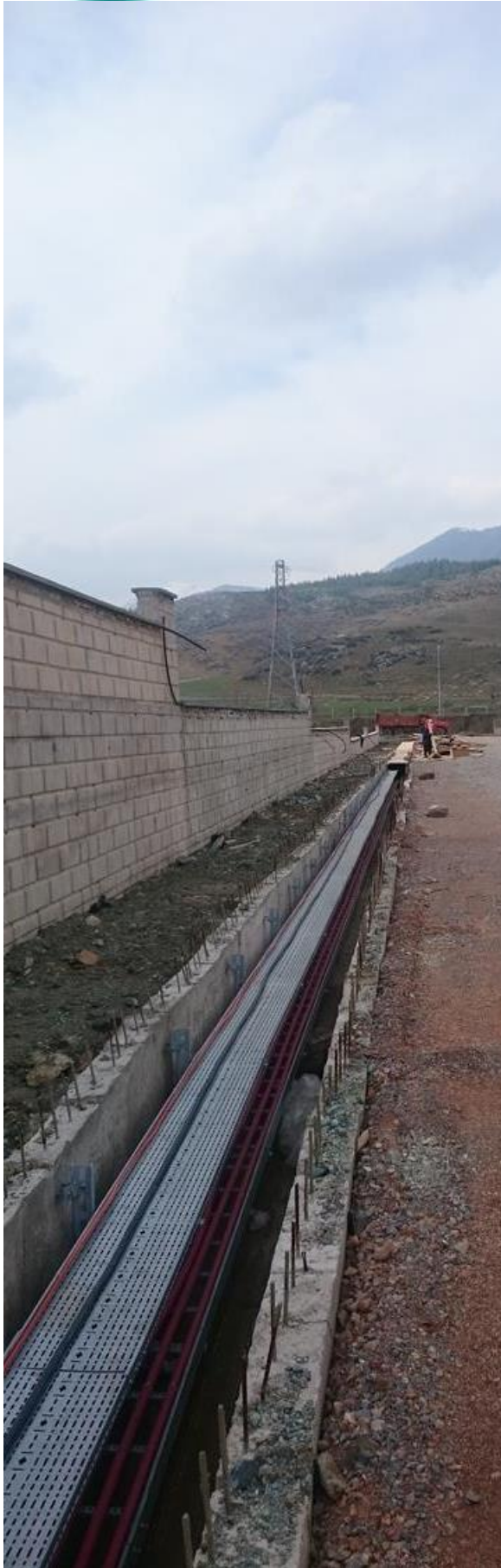
Cable Pull to Cable Tray
