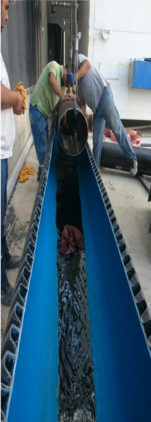
Pipe Cleaning with Special Chemicals
